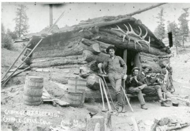
Figure 15. The cabin of S. J. Roberts (possibly the man standing). These young men, seen with a fife and fiddle, likely owned a mine they were developing themselves during the early days of the gold camp. The tools, rope, and wooden buckets were used to dig a shaft. Photo date August 1893 by W. J. Gillen. Courtesy of the Cripple Creek District Museum.
