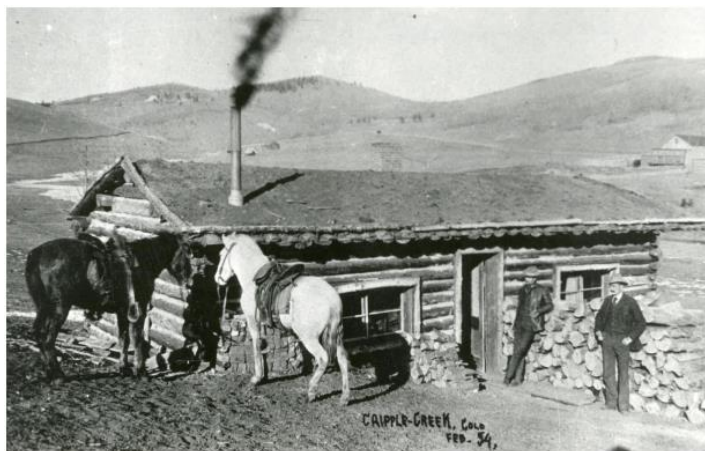
Figure 17. Spencer Penrose and Charles L. Tutt stand in front of their one-story log cabin with a low gable and sod roof. Two saddled horses are tied to the corner of the cabin. Penrose and Tutt built the cabin in 1891. Photo date February 1894 by W. J. Gillen. Courtesy of the Cripple Creek District Museum.
