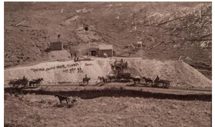
Figure 13. Chicago Cripple Creek Tunnel, Cripple Creek. The Chicago tunnel enters Globe Hill from Poverty Gulch, a short distance east of the Abe Lincoln mine, and
